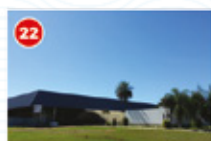
Expo Pavilion in the City Park
